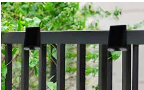
Cable tie installation
